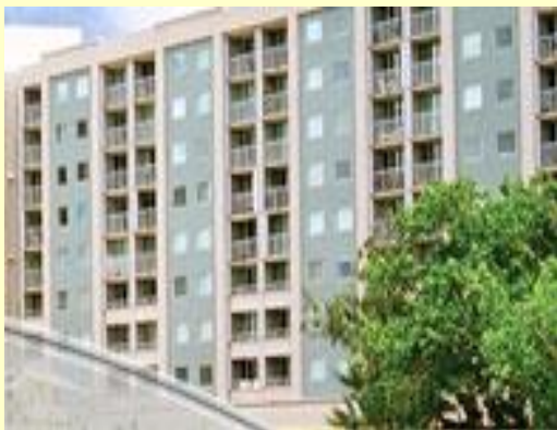
Alupang Cove Condominium Exterior Wall Replacement Project
