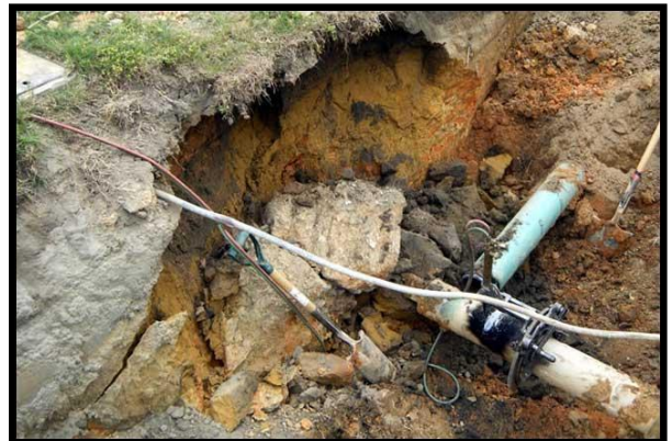
The trench collapse photos from different angles.
