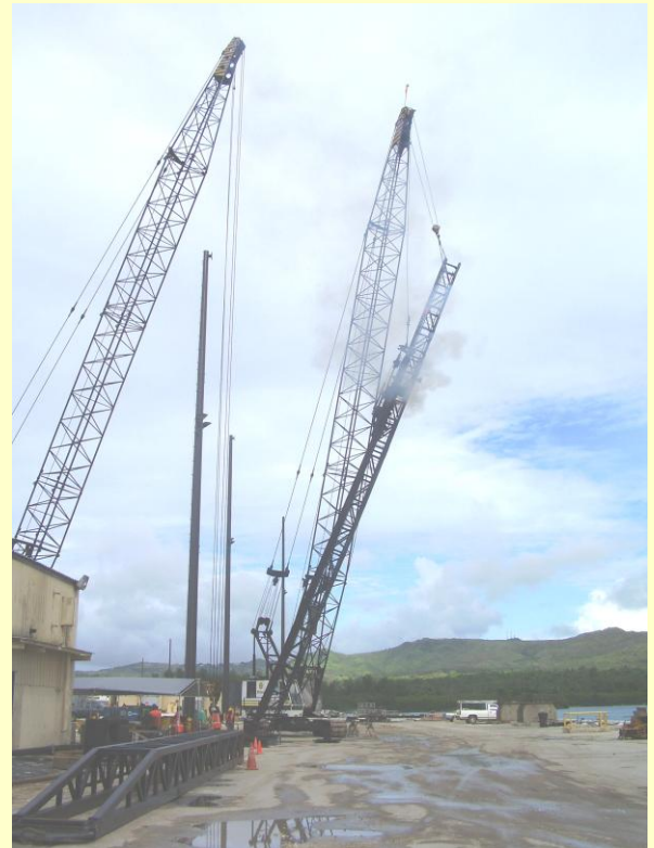
"Last Pile Being Driven"
